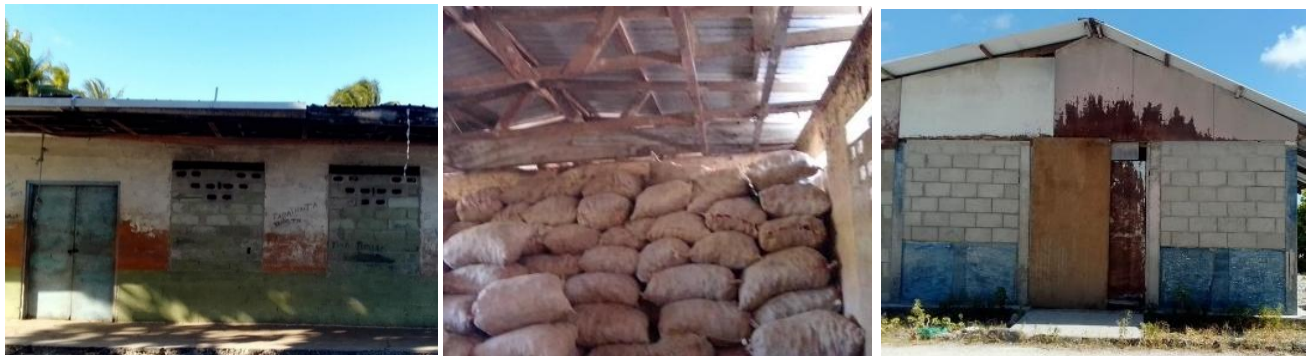
Source: Copra sheds on Nikunau captured by the audit team in May 2025
